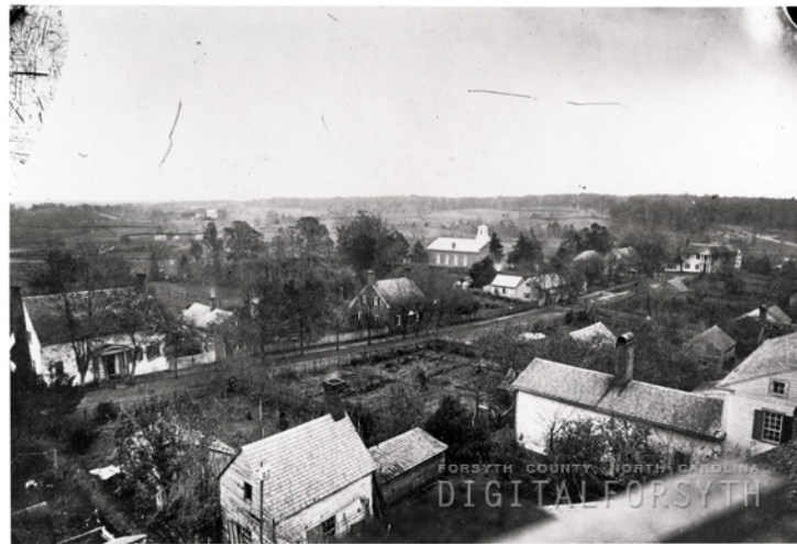
Figure 1. This circa 1866 photograph shows Church Street in Salem, North Carolina. The old African American Moravian log church, built in 1823, can be seen near the center of the image -- it's a small building with two chimneys. The updated brick church, built in 1861, can be seen to the right and behind it, with a white roof and bell tower.
